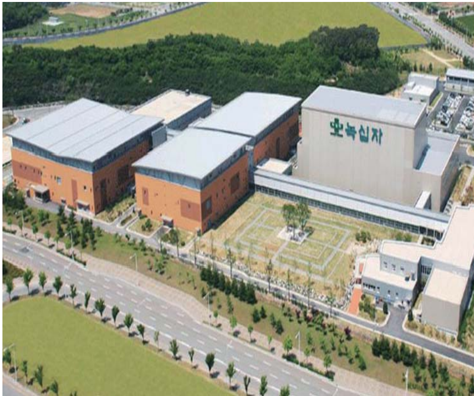
Blood Preparation Plant of Green Cross in Thailand
